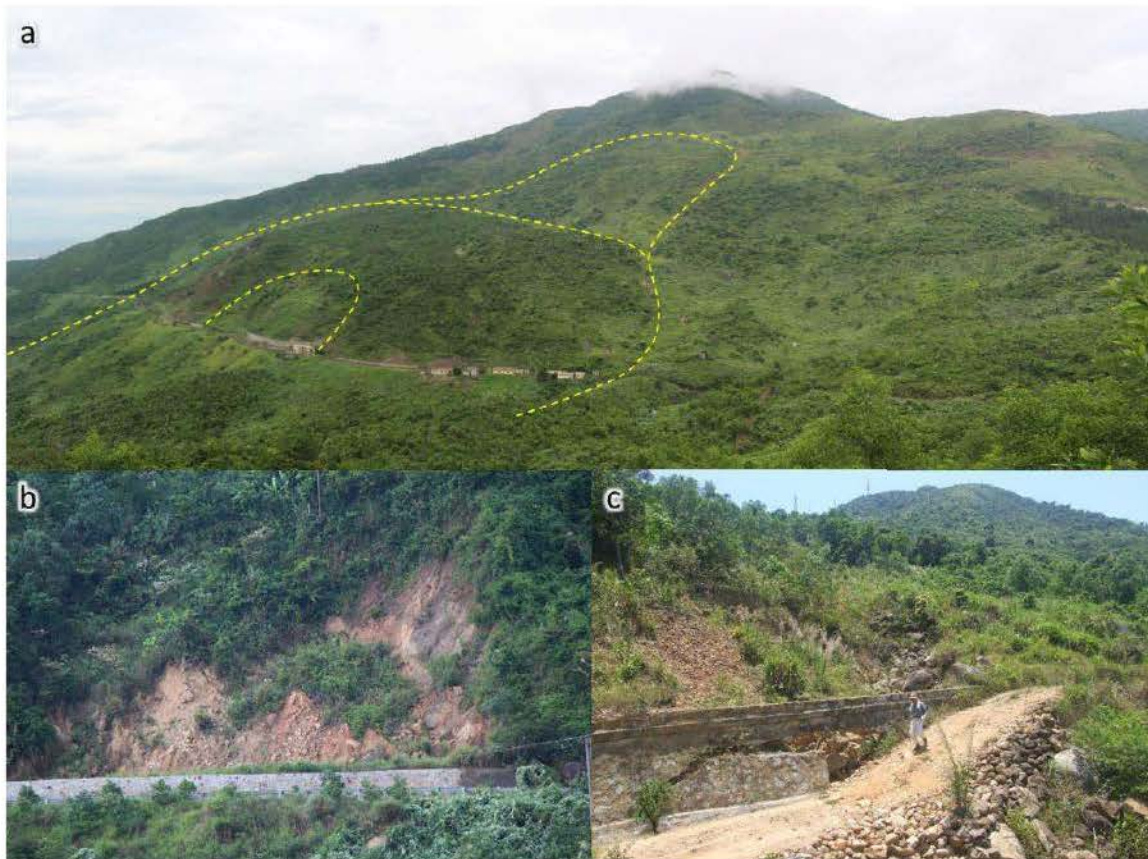
Figure 2.12 Some landslide at Hai Van (a, photograph by Dinh; b, Tien et al., 2015; c, photograph by Le): a: overview landscape of old landslide at Hai Van railway station; b: rotational slide; c: landslide damaged retaining wall
