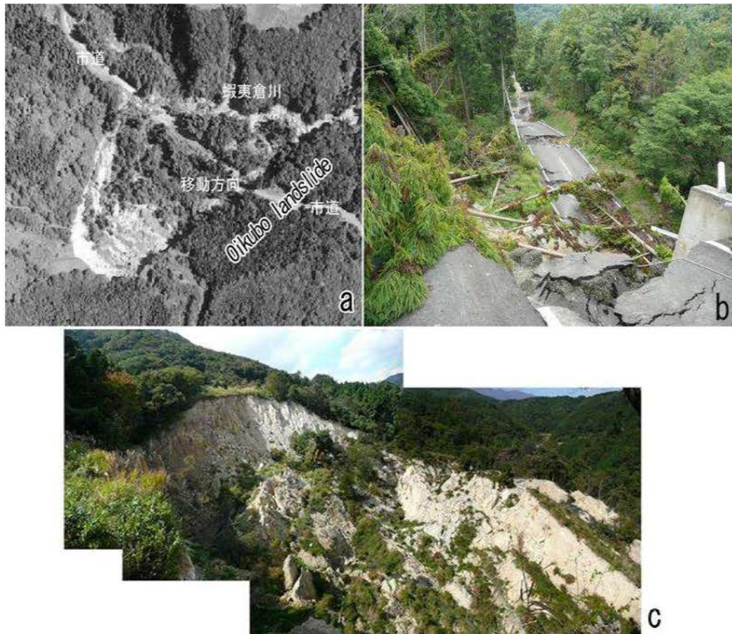
Figure 3.16 Oikubo landslide (a: aerial photograph after the movement; b: prefectural road cut and transformed about 30 m; c: overview of the upper part of landslide (Higaki et al., 2008)
