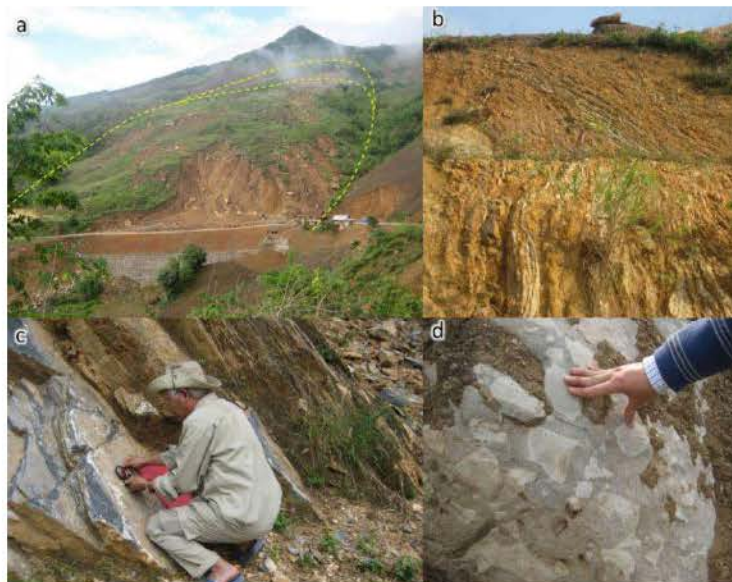
Figure 2.3 Landslide at Km 447+900, National Road No. 37 (taken by Vinh, 2009): a: overview of landslide; b: sedimentary rock bedding was bent because of intruded basalt; c: bedding plane parallel to slope; d: conglomerate
