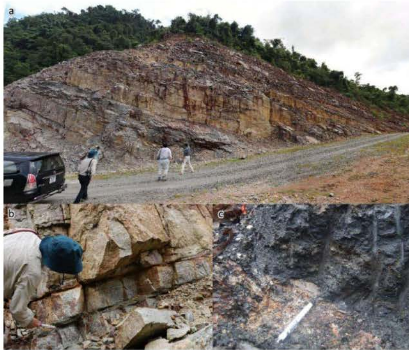
Figure 2.10 Typical geology structure of Song Bung Pass (Le et al., 2015a and 2015d): a: well bedded layer structures; b: some weak layer between sedimentary rocks; and c: lenses of coal layer, it is also a slip surface.
