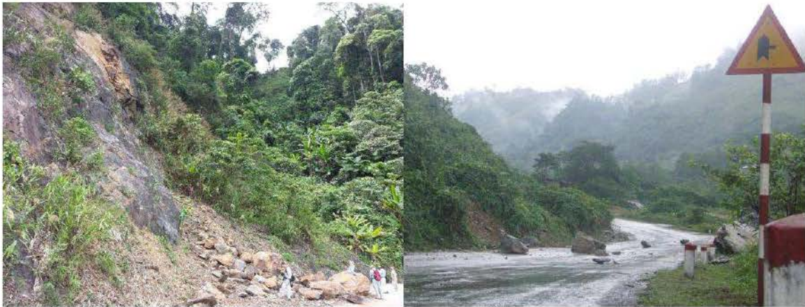
Figure 3.27 Rock fall (photograph by Le)
