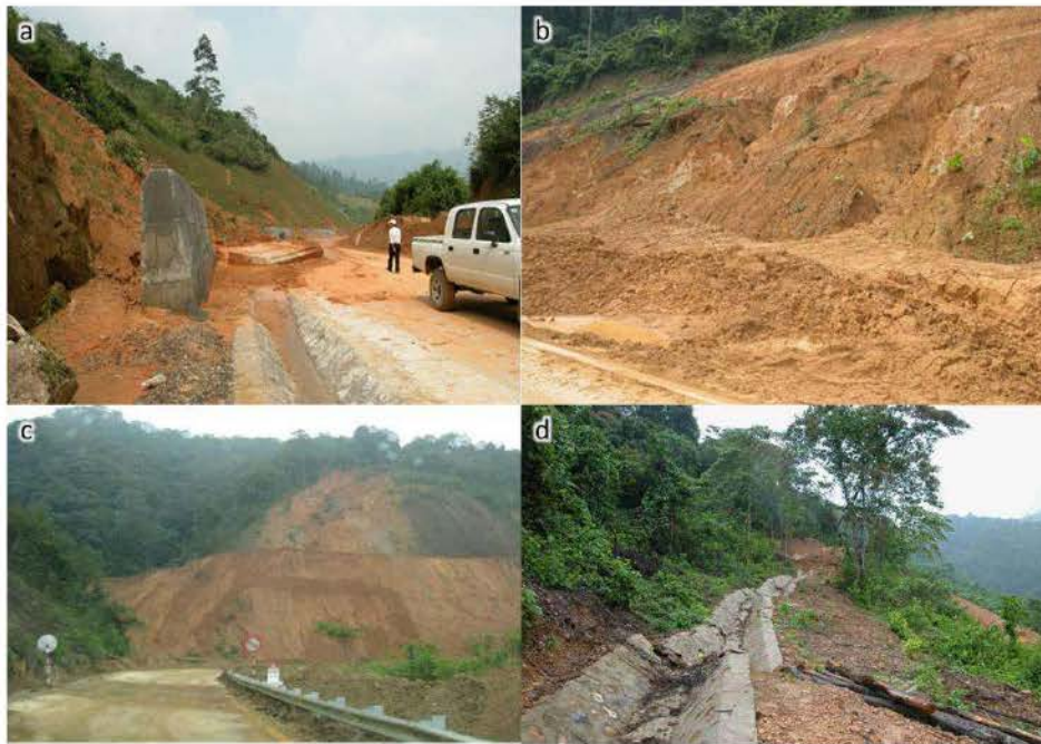
Figure 2.9 Typical landslides in Ho Chi Minh route (2) (Doan, 2008): a, b: debris slide at Km 339; c: rotational slide at Da Deo Pass; and d: rotational at Km516+713 damage ditch at upper slope. These landslides reactivated after a period of heavy precipitation
