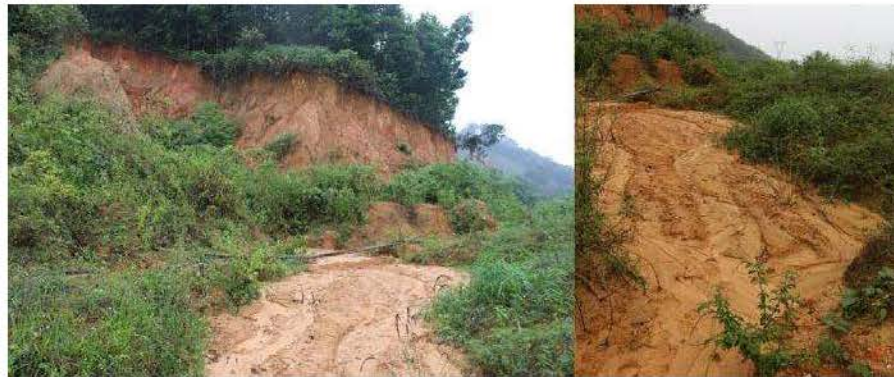
Figure 3.30 Debris flow (photograph by Le)
