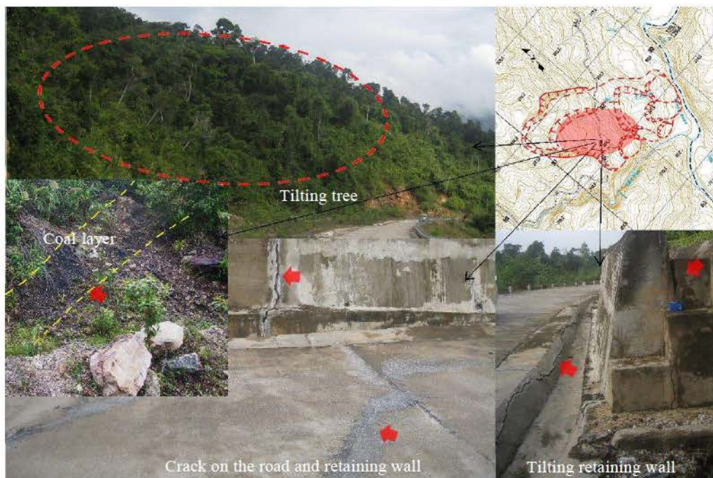
Figure 5.12 Some evidence of landslide action was observed at a part of landslide No. 18 (Le, 2015a)
