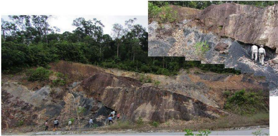
Figure 3.29 Translational slide (photograph by Le)
